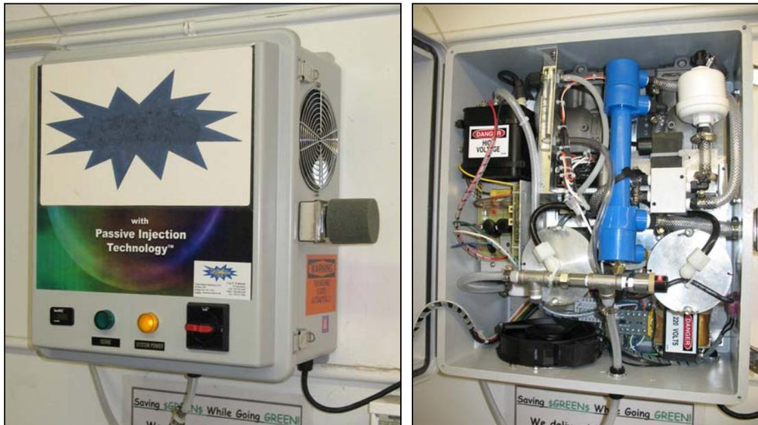
**Figure 2.** Ozone Generator Mounted on Wall of Laundry Room (L) and With Cover Open (R)
